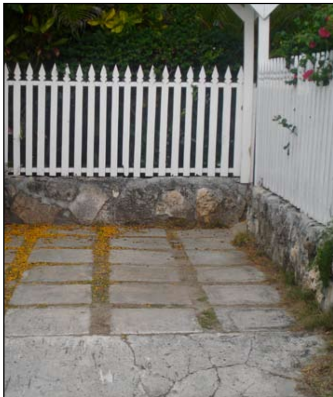
T4: Stone Paver Golfcart Parking, Dunmore Street
