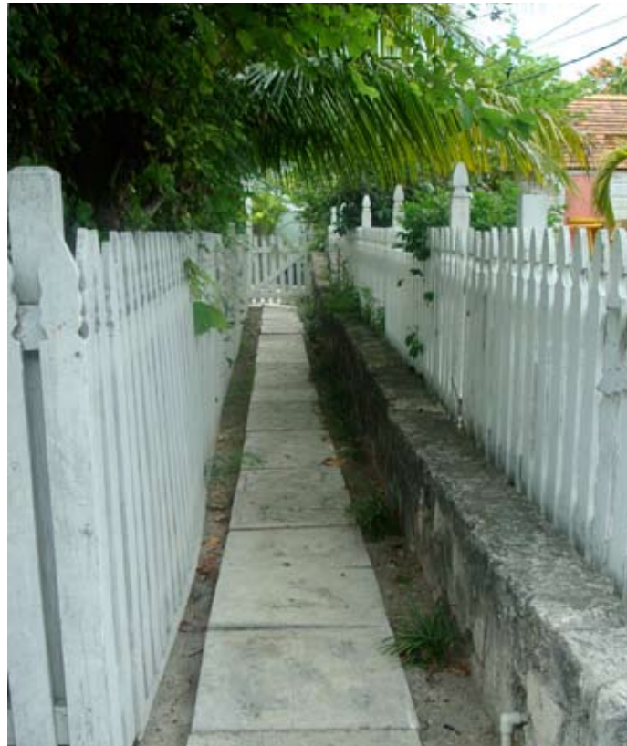
T5: Concrete Pavers, Near Temperance Square
