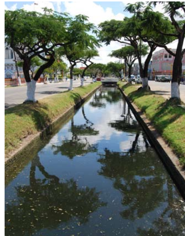
GEORGETOWN, GUYANA: Drainage infrastructure as civic art
