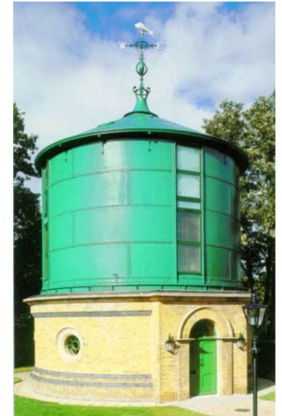
WATER TOWER: Possible precedent
