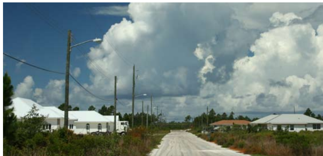
SANDY POINT: Some existing ranch houses
