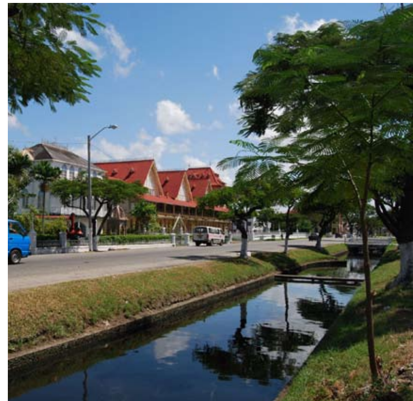
GEORGETOWN, GUYANA: Drainage infrastructure as civic art
