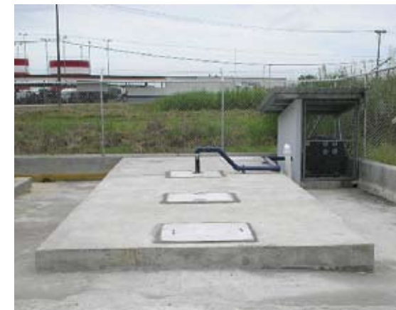
FAST SYSTEM: Shown after installation
