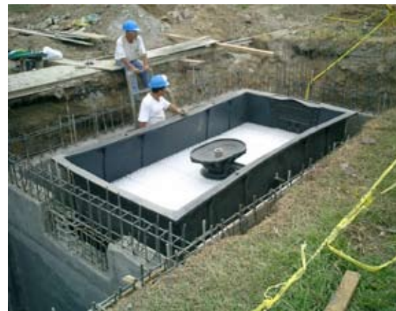
FAST SYSTEM: Shown during installation
