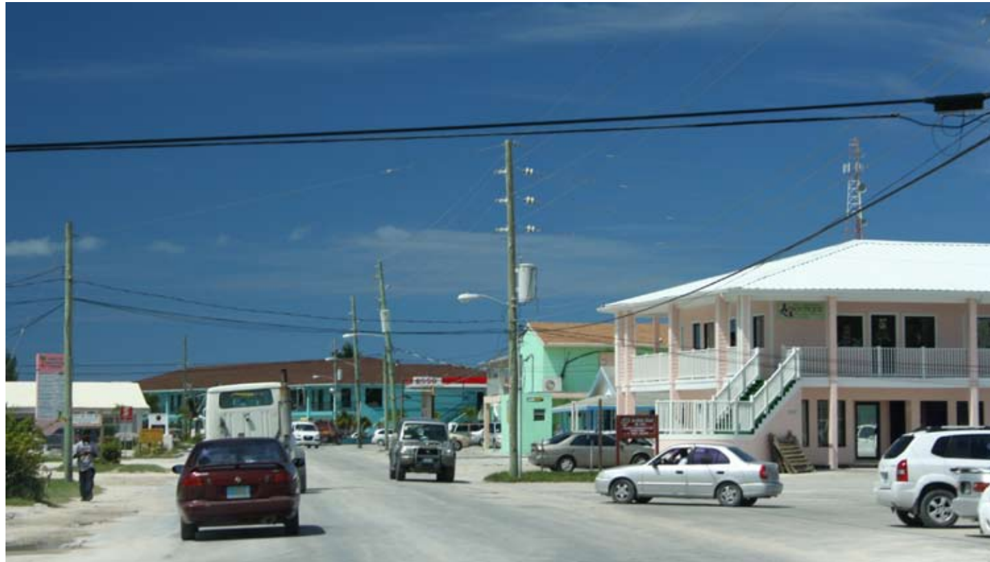
MARSH HARBOUR: Don McKay Boulevard, looking north
