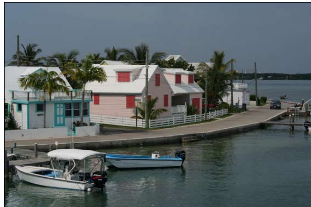
SPANISH WELLS: Small blocks provide frequent access to important places.
