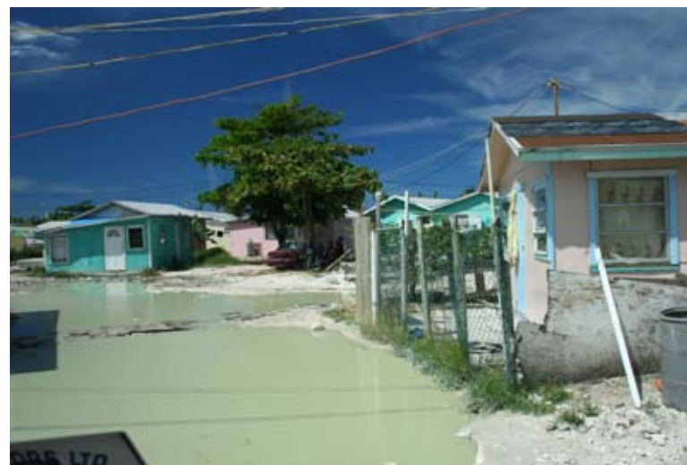
ROUTINE STREET FLOODING
