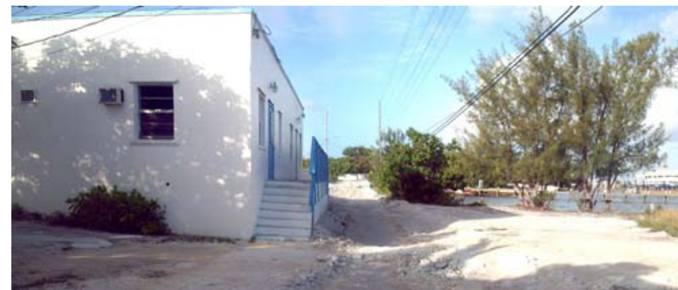
ALBURY BOULEVARD: Existing view looking west
