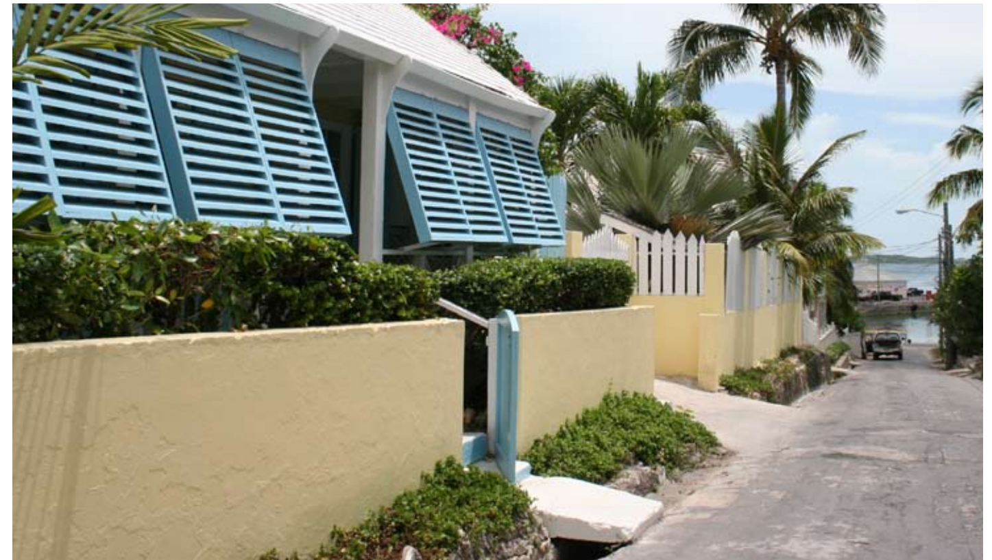
T5: Open Gutter with Bridges, Murray Street
