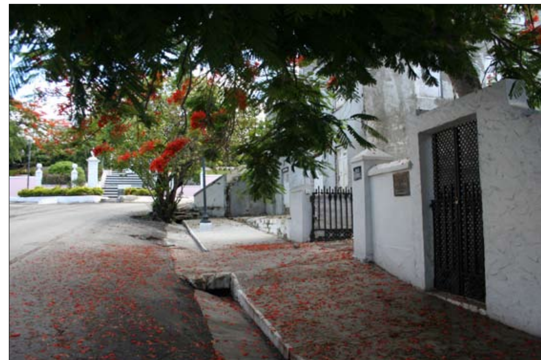
NASSAU: Traditional open gutters can help to channel stormwater to light imprint detention and retention areas.
