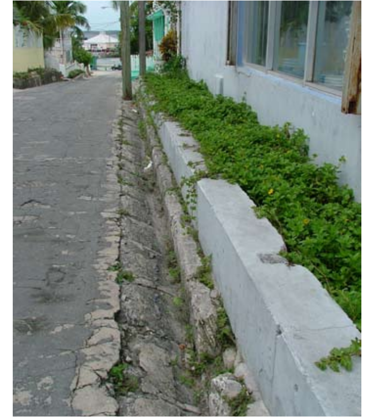
T5: Open Gutter, Murray Street
