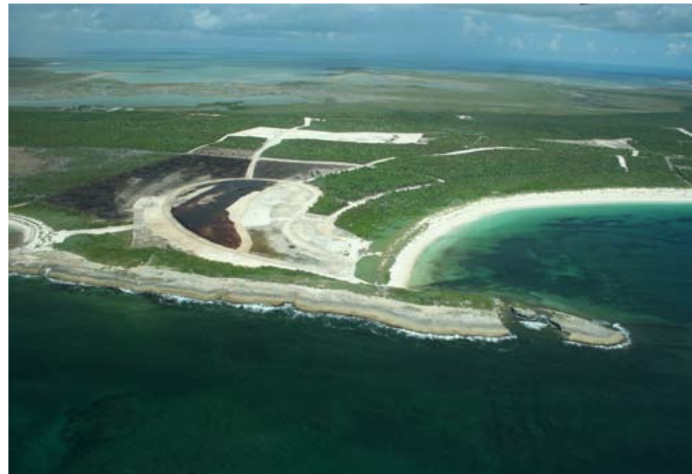
SCHOONER BAY: Under construction in July 2008
